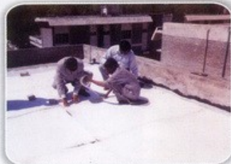
Joining insulation rolls with jointing strip
