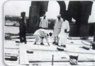
Laying of reinforced concrete over 2" Diamond Jumbolon-Rolls at Serena, Islamabad
