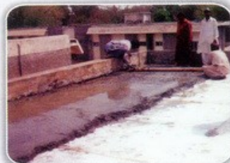
Laying of plain concrete over Diamond Jumbolon-Rolls, in panels of 4' x 4' with 1/2" deep false joint
