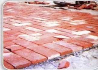
Fixing of tiles and cement mortar
